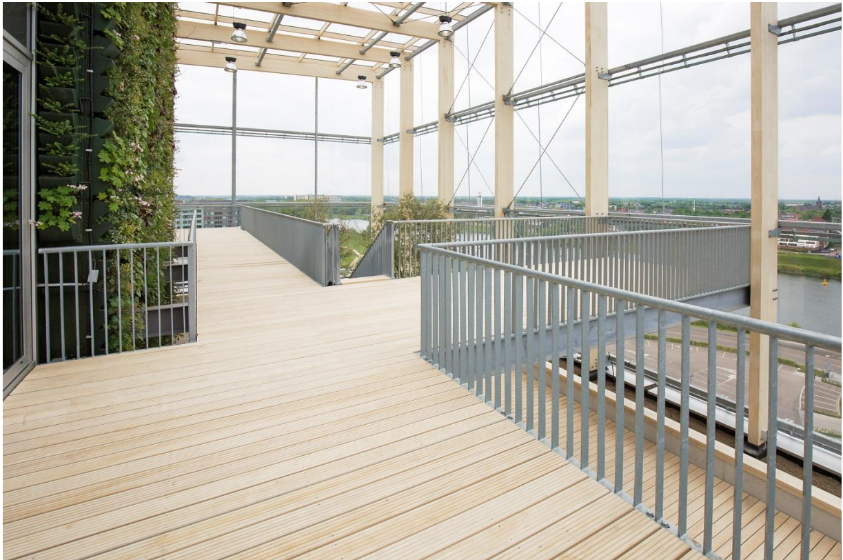
Accoya was specified for Venlo City Hall, NL. This building boasts the highest possible application level of Cradle to Cradle
